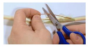
Using the same OGCL stripping tool the cable jacket will also need to be opened at the location where the Demarcation Box will be installed.
