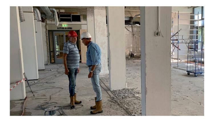
Andreas Reckers, Sales Manager at Nexans, explains: "A key advantage of this design approach was the fact that no major structural alterations were required. We could also realise significant savings in terms of available floor space, wall penetration, and pipe routes. We replaced several backbone cables and hundreds of copper cables, which were managed from several distribution rooms, by just forty OM4 fibre optic cables and forty zone distribution boxes."
